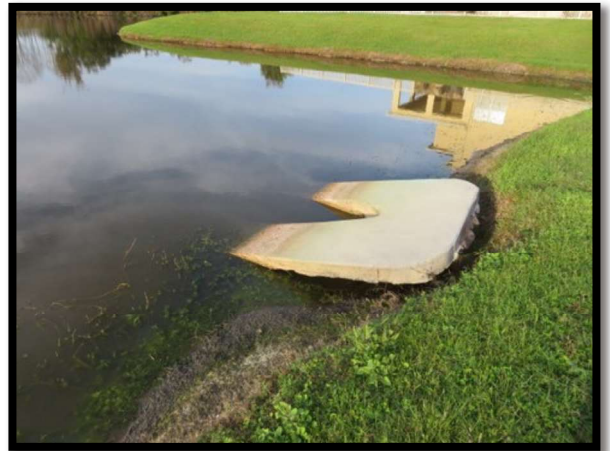
Figure 18 Pond 34 Shoreline Erosion
