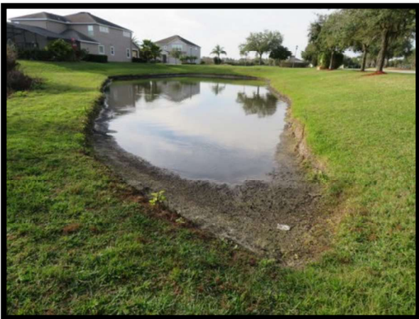
Figure 15 Pond 3 Shoreline Erosion
