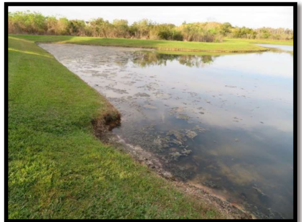
Figure 18 Pond 34 Shoreline Erosion
